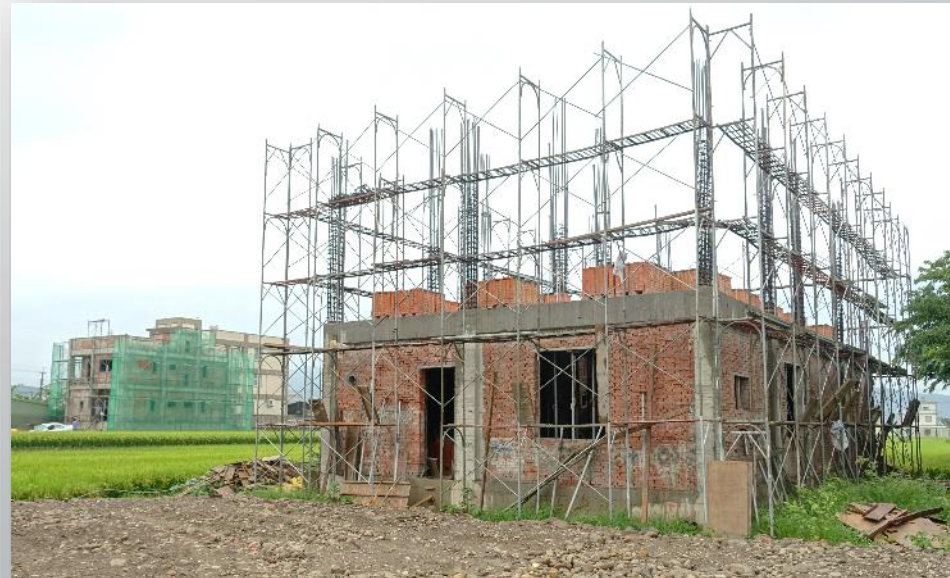
Second home construction, Gongguan
